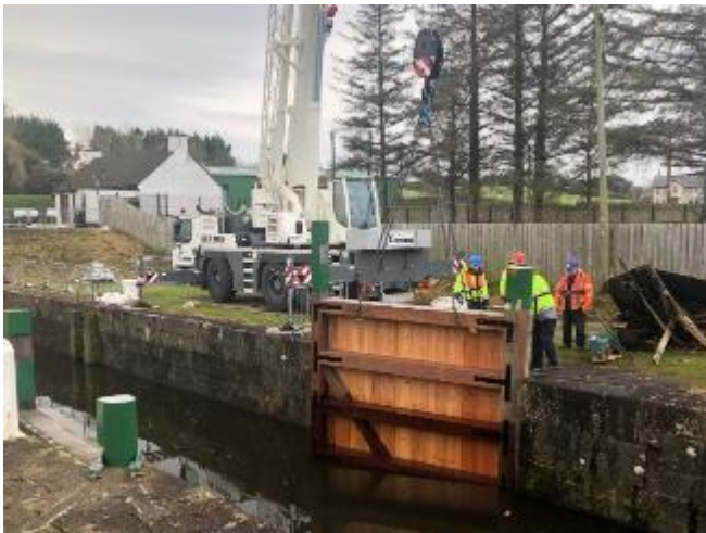
Portna Lock Gate Repair and Replacement, Lower Bann
