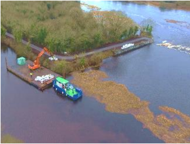
Towpath Works at Meelick Weir
