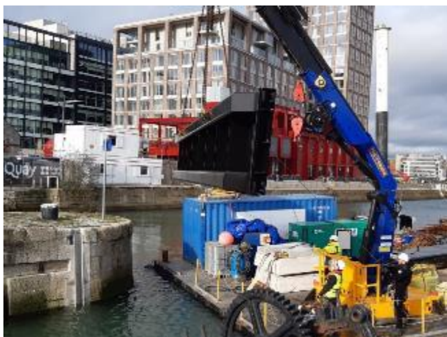
Camden Lock Installation of Removable Steel Stop Logs
