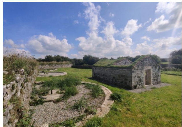
Conservation works at Fort Eliza on the Shannon
