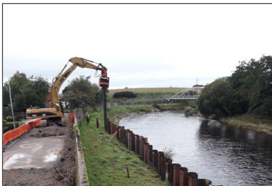
Hunters Crescent Omagh - Floodwall Replacement Scheme Under Construction
