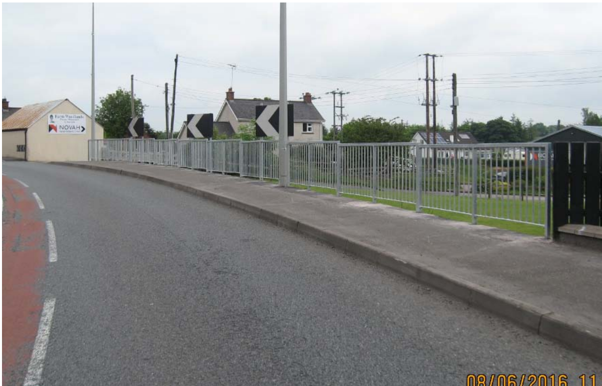
New Pedestrian Guard Rail on A4 Crossowen Rd Augher
