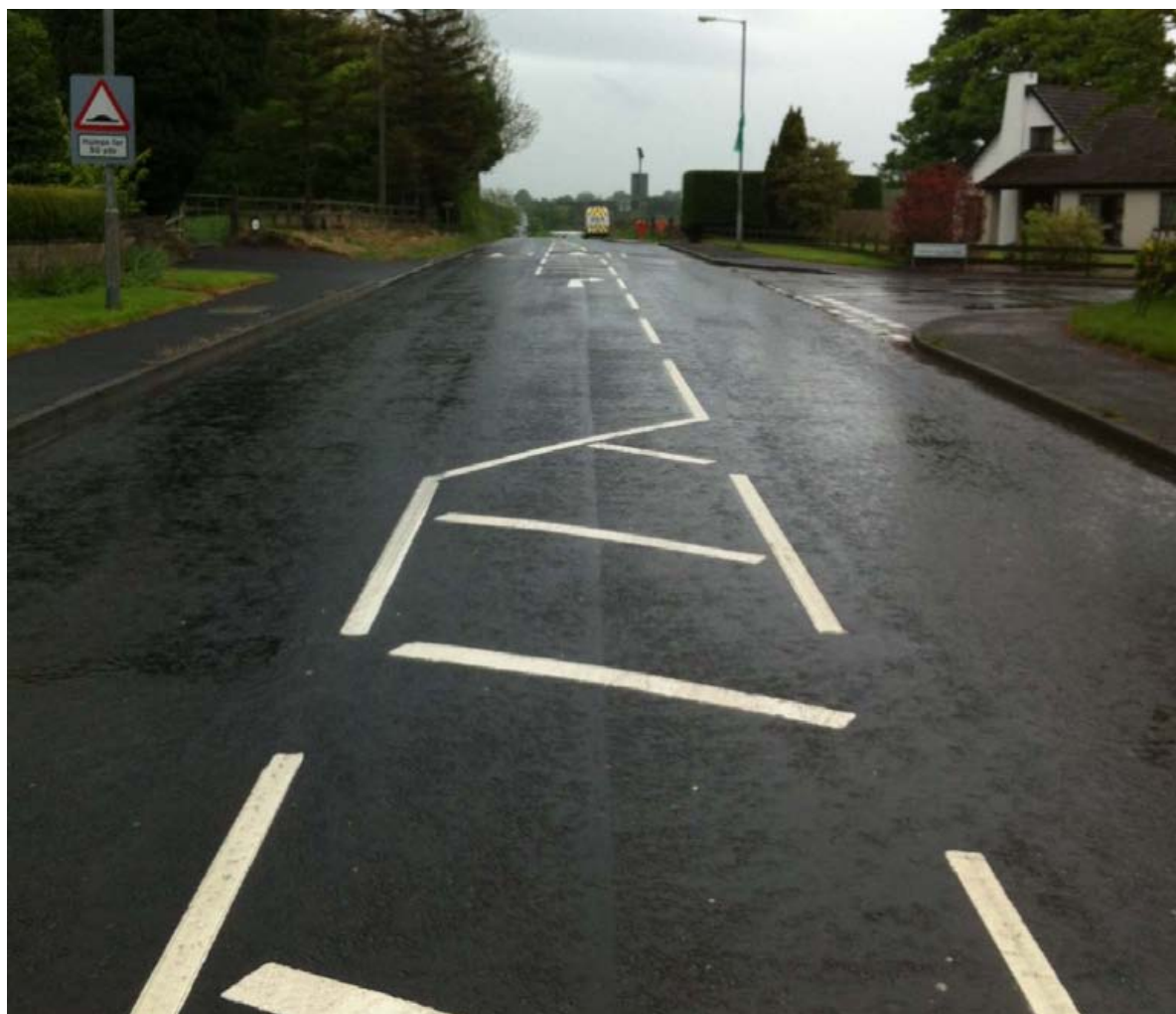
Resurfacing of B40 Magherafelt Road Draperstown
