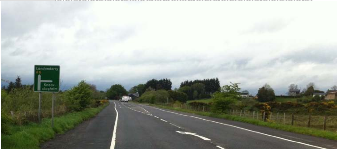
Resurfacing A6 Glenshane Road at Derganagh
