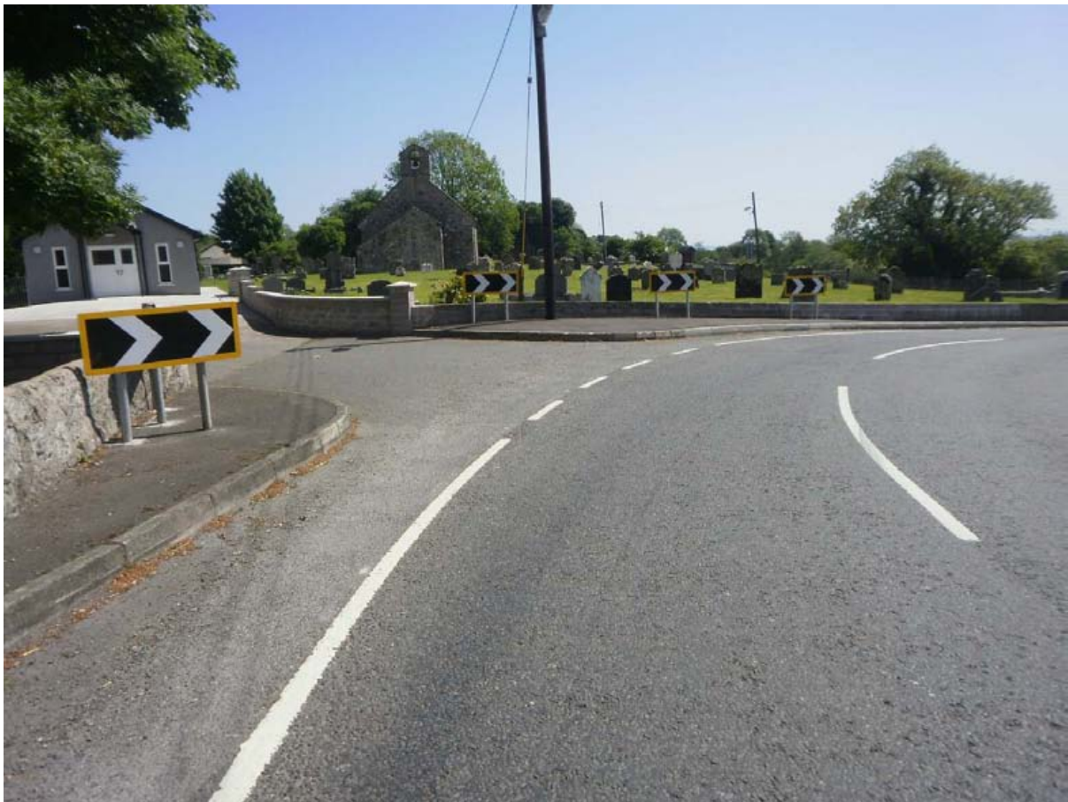
Upgraded bend warning signage on Mountjoy Road at Clonoe Parish Church
