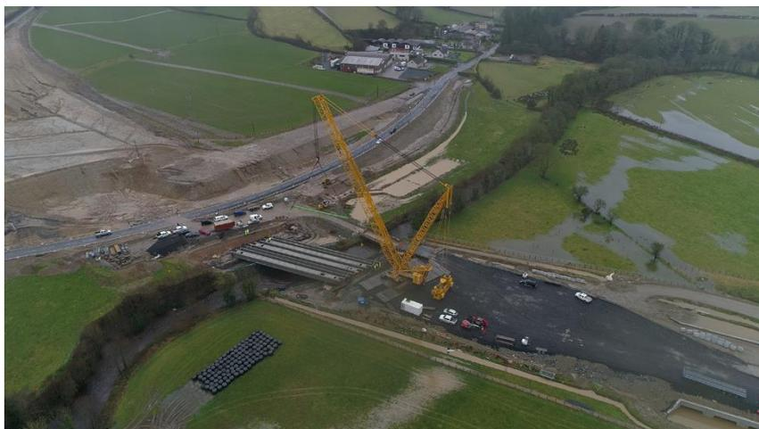
**Beams being installed on the Owenreigh River bridge**
