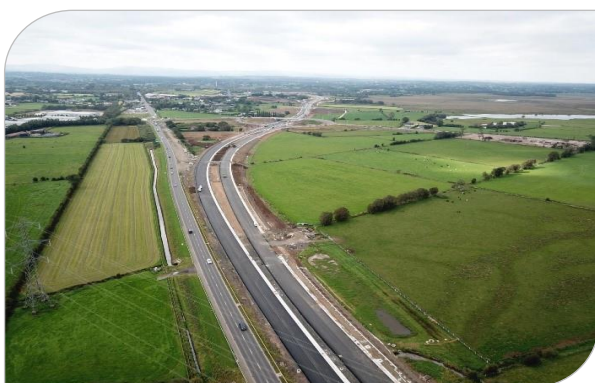
Aerial view looking west Toome Bypass tie-in
