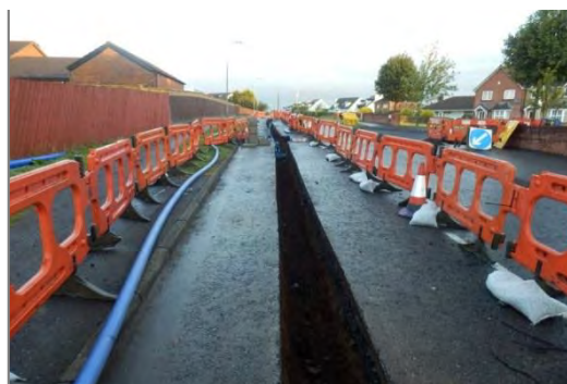
Figure 2.7: New mains installation
