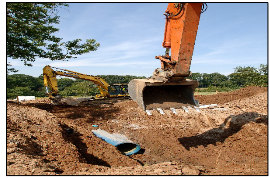
Figure 2.7: New mains installation
