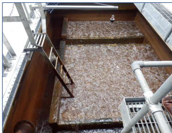
Figure 2.2: Backwashing a Filter
