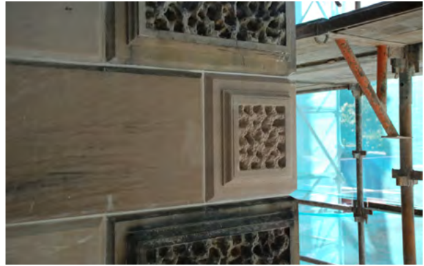
Above left: Inappropriate mortar repairs can exacerbate erosion of original stonework and compromise the essential character and appearance of historic buildings. Above Right: Removal of defective mortars and repairing with stonework and detailing to match the original, conserves the buildings architectural interest.
