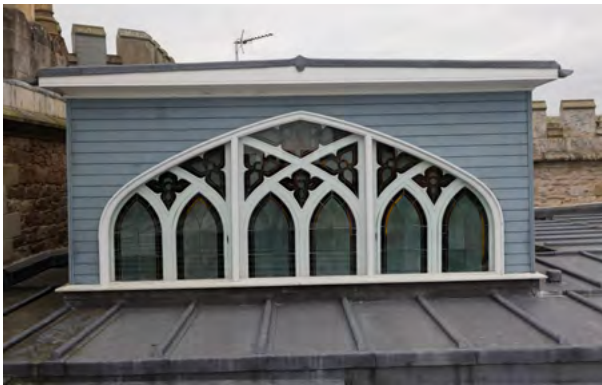
Above: Killymoon Castle, Cookstown: Before, During & After. Replacement of a defective lead roof revealed the underlying timber roof structure around the central cupola, which informed the conservation repair approach to a key feature of special interest. A new replacement lead roof has safeguarded the ornate cupola and underlying building fabric.
