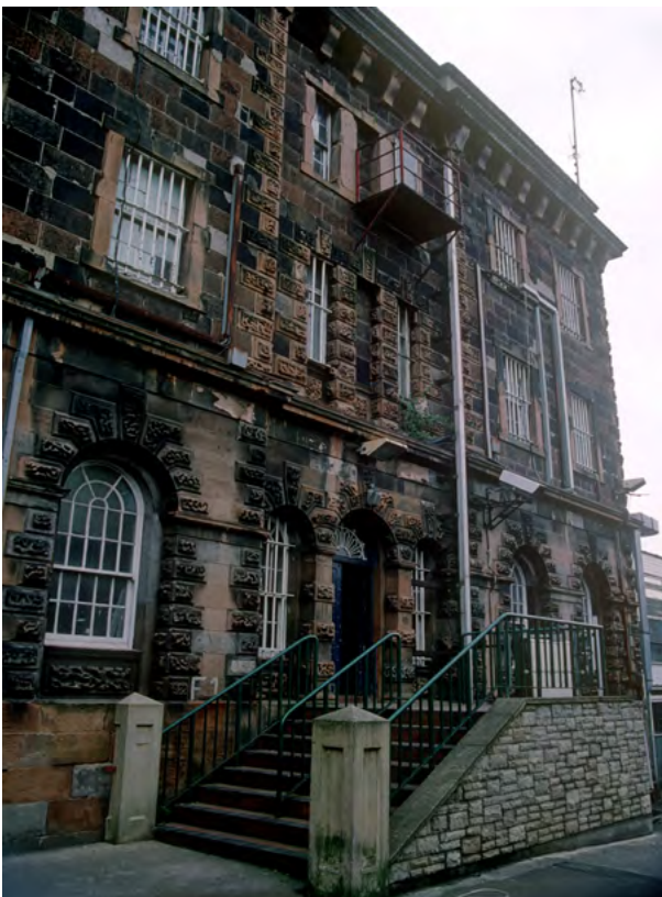
Crumlin Road Gaol, Belfast. Historic records informed the sympathetic design and layout of the new replacement steps incorporating concealed lift access, in keeping with the architectural design and character of the building.
