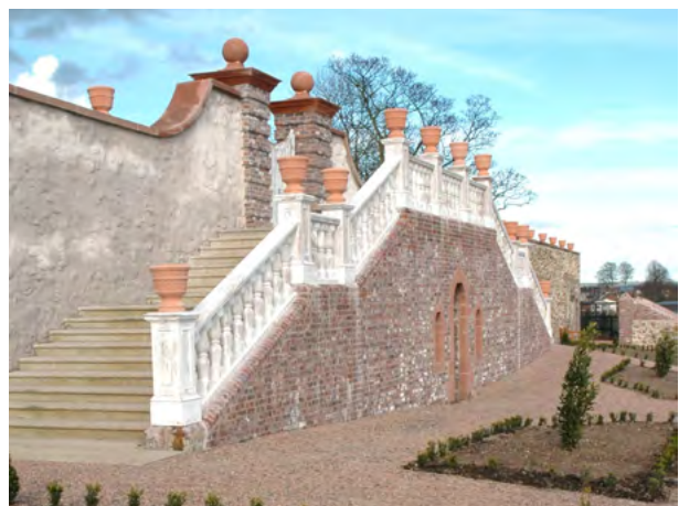
Above: Lisburn Castle Gardens: Before & After: Excavation works informed conservation and presentation of castle gardens.
