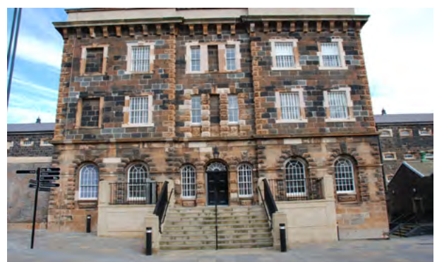
Crumlin Road Gaol, Belfast. Historic records informed the sympathetic design and layout of the new replacement steps incorporating concealed lift access, in keeping with the architectural design and character of the building.
