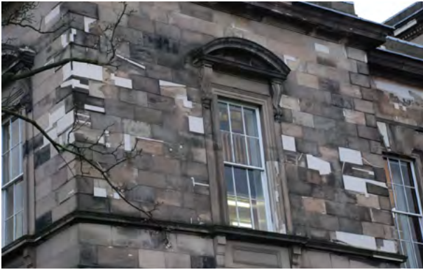
Above left: Inappropriate mortar repairs can exacerbate erosion of original stonework and compromise the essential character and appearance of historic buildings. Above Right: Removal of defective mortars and repairing with stonework and detailing to match the original, conserves the buildings architectural interest.
