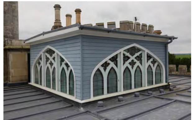
Above: Killymoon Castle, Cookstown: Before, During & After. Replacement of a defective lead roof revealed the underlying timber roof structure around the central cupola, which informed the conservation repair approach to a key feature of special interest. A new replacement lead roof has safeguarded the ornate cupola and underlying building fabric.
