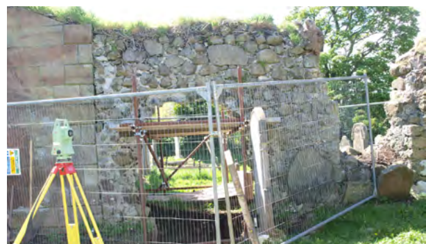
Above: Templecorran Church, Ballycarry: Excavations to inform consolidation of a doorway.
