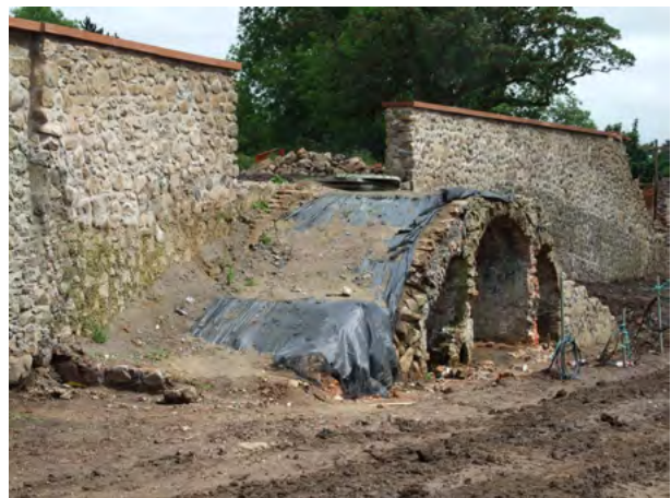
Above: Quoil Castle: Excavations at 1st floor to inform consolidation of cracked vault.
