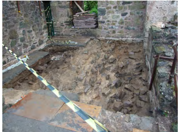
Above: Quoil Castle: Excavations at 1st floor to inform consolidation of cracked vault.
