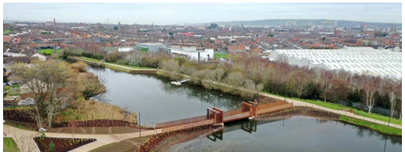
An aerial photo of the work completed to date at Springfield Dam.
