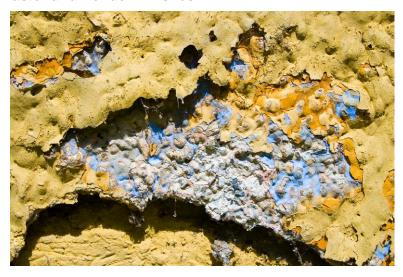
One of the first tasks may be to remove inappropriate materials and methods of repair and replace with the appropriate stucco/render. However, removal should only be carried out if this does not put greater risk on the original fabric. It may also be necessary to cut out defective areas of the original that cannot be saved.
