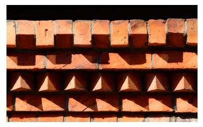
When pointing is contemplated, joints should be raked out to a depth of 25 mm and repointed using a lime: sand mortar. Joints are to be finished flush or slightly recessed from the adjoining brick faces. As it can be damaging to the adjacent brick arrises to remove well-adhered cement mortar, it is often better to avoid removing sound cementations pointing. Where cracked and open, carefully remove cementitious mortar with fine masonry chisels avoiding power tools.
