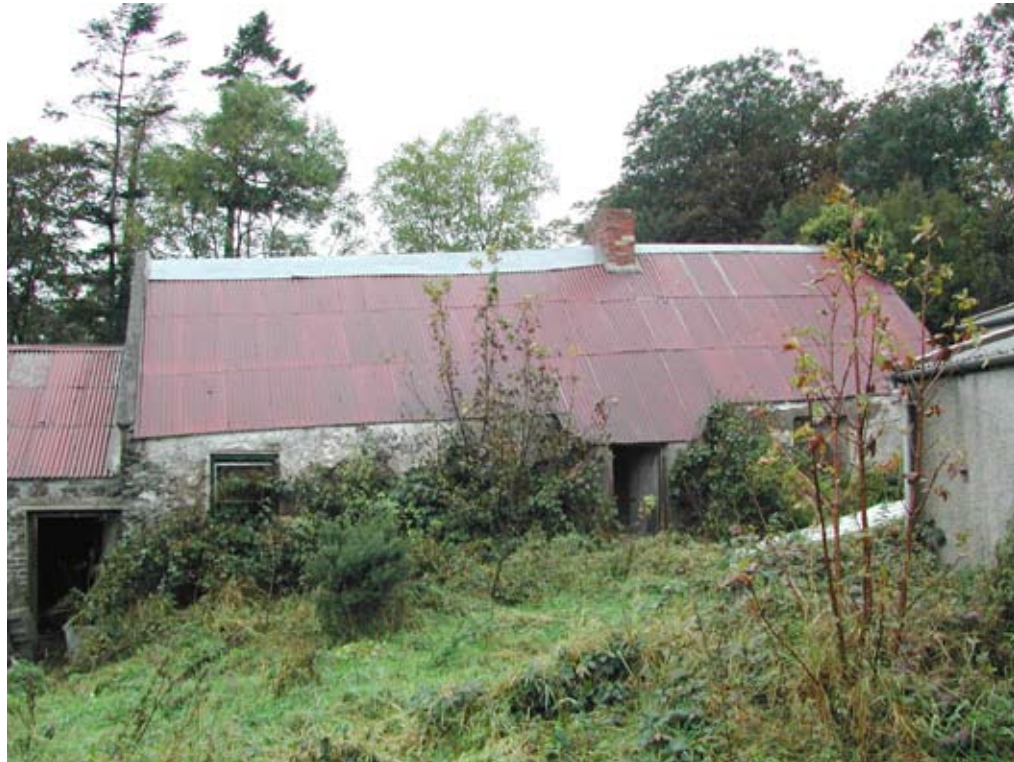
Magherabally Cottage before restoration and (right) after.
