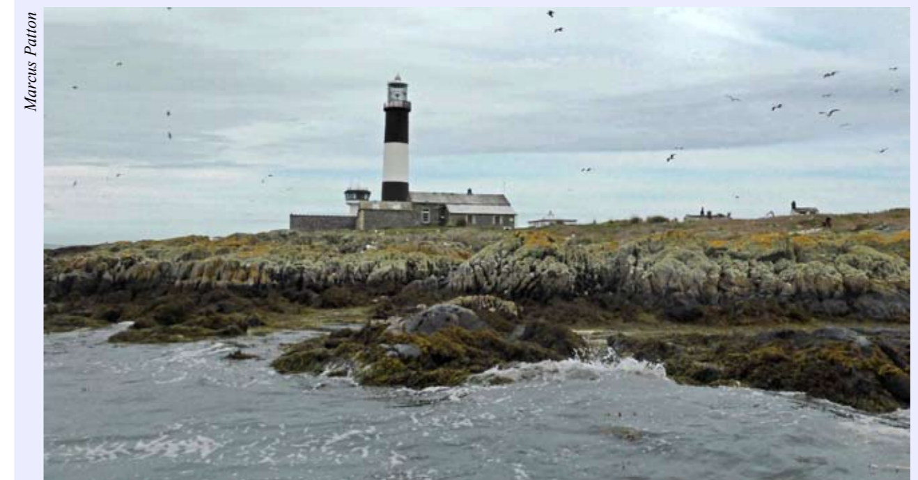
One of the most unusual buildings listed this session was Rathlin West lighthouse ( above ). Instead of the conventional pillar surmounted by a light, the lighthouse is quite a classical six-storey building and the light is "upside-down", set below the house so as to be more visible from the sea than if it had been built at the top of Rathlin's cliffs.
