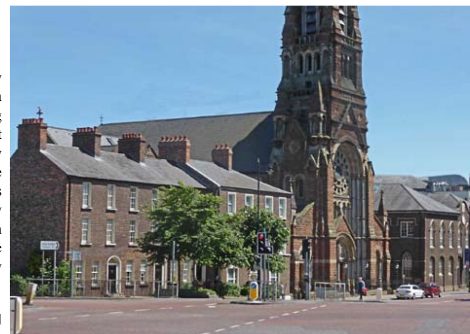
Donegall Street, Belfast: historic buildings at risk restored as social housing.
