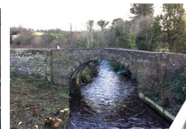
(above) Burntollet Bridge before its demolition.
