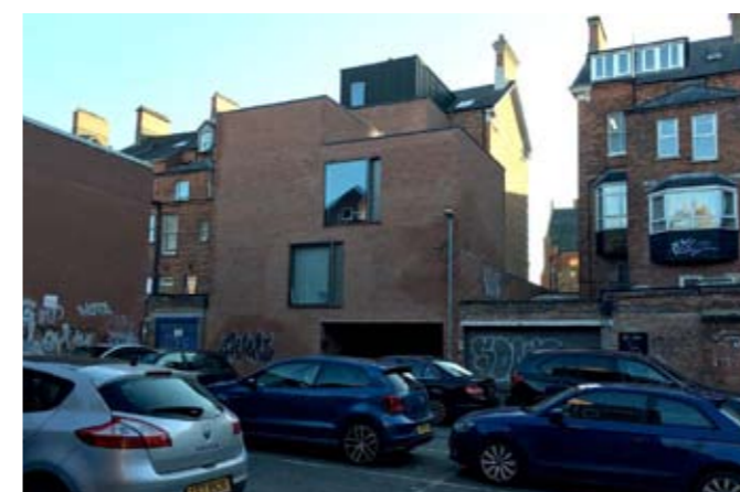
College Gardens extension (above) and front elevation (facing page)
