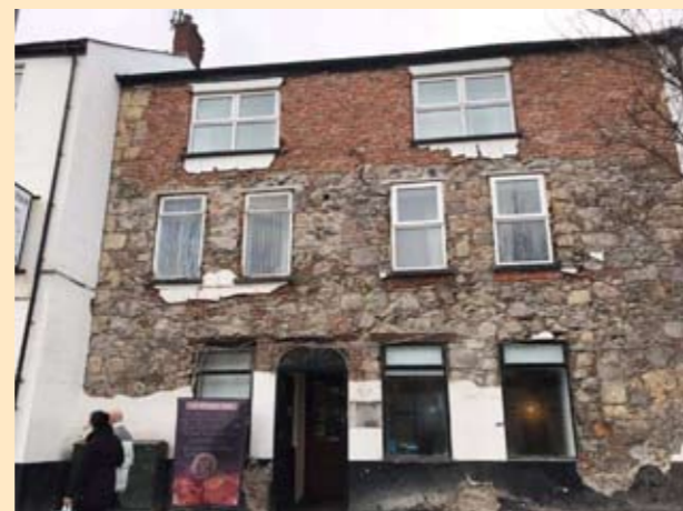
Dobbin's Hotel (above) as it was in the 1960s, a Victorian frontage with widened second floor windows; then during the works, with the render stripped off to reveal two storeys of rubble stonework and a later second floor; and (bottom) the rediscovered castle, with conjectural castellations and modern windows.
