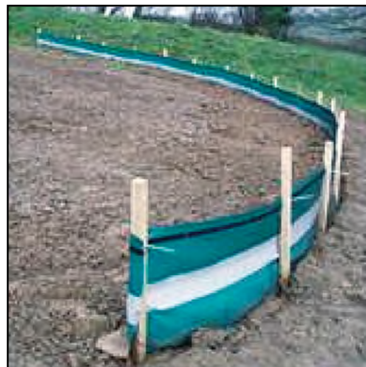
Photo 22 - Sediment fencing
