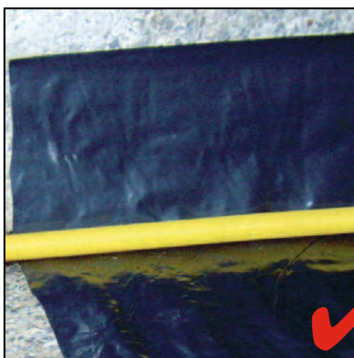
Photo 9 - Protecting silage pit wall-floor joints
