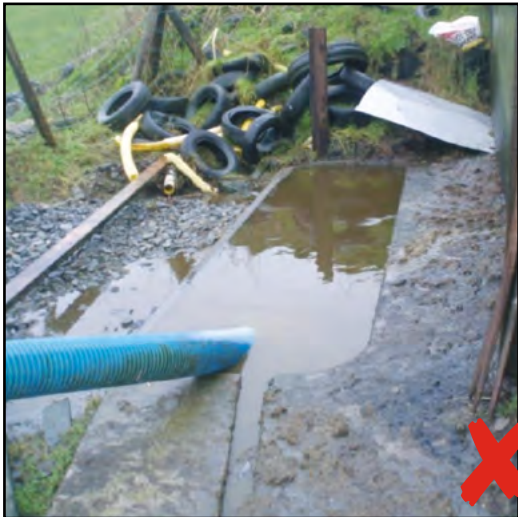
Photo 12 - Overflowing effluent tank not being managed
