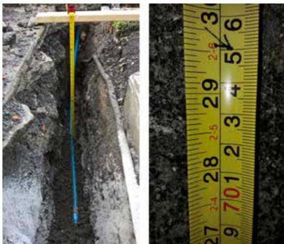
The pipe should be laid in a bed of quarry dust or pee gravel. The pipework entering the building should be passed through a duct and sealed at both ends and insulated. We have to inspect this when the ground is open.
