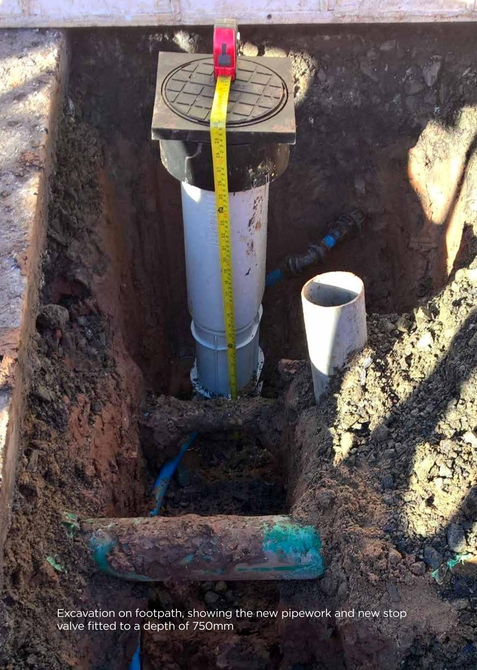
Excavation on footpath, showing the new pipework and new stop valve fitted to a depth of 750mm
