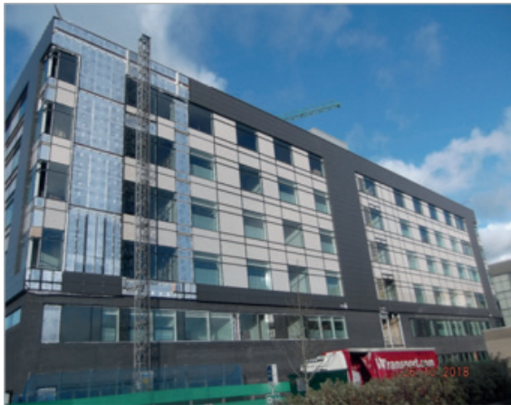
Acute Services Block completing south façade
