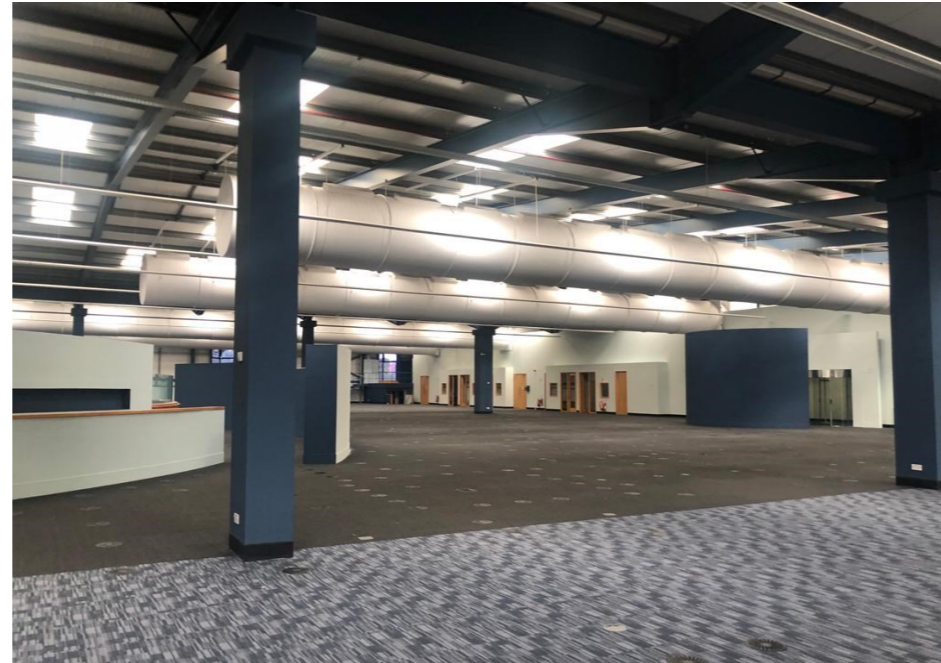
Figure 26: Inside Telettech Building
