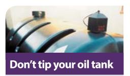
If you tip your oil tank you risk damaging the pipe, whilst dirt disturbed at the bottom of your oil tank may enter the heating system and cause further serious damage.
