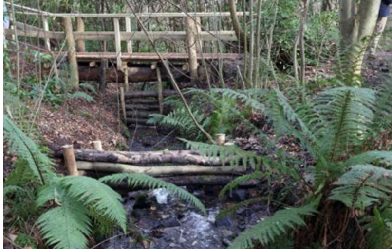
The 'leaky dam' which helps control the flow of flood water
