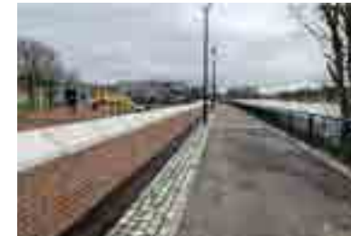
Brick-clad reinforced concrete flood wall with anti-climb coping
