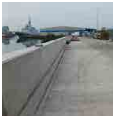
Flood wall under construction in Belfast Harbour
