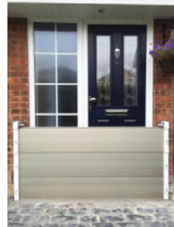
Flood gates can prevent or slow the ingress of flood water
