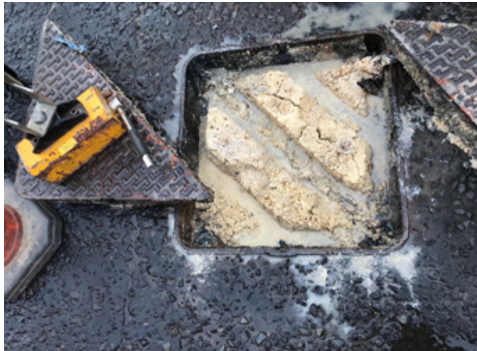
L to R: removing rubbish from a domestic drain; Main sewer blocked with Fatberg; The process of clearing a Fatberg
