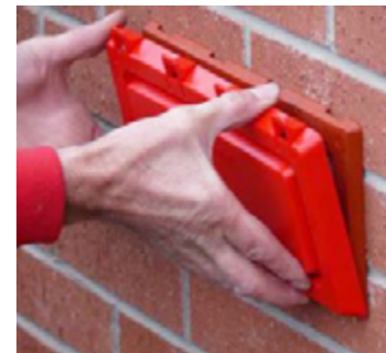
Plastic covers can stop flood water entering through airbricks
