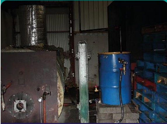
Photo of fuel laundering equipment
