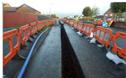
Figure 2.8: New mains installation
