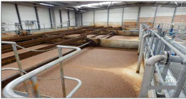
Figure 2.2: Flotation Stage
