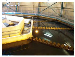
Figure 2.2: Backwashing a Filter
