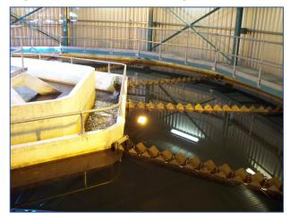
Figure 2.2: Backwashing a Filter
