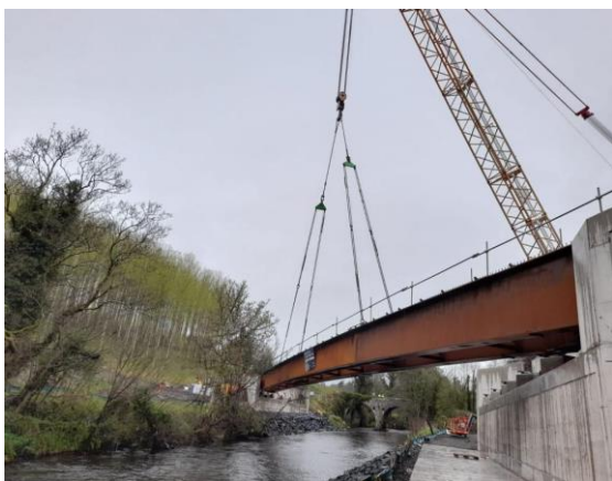
Beams being lifted in place for the Ardmore Road bridge.
