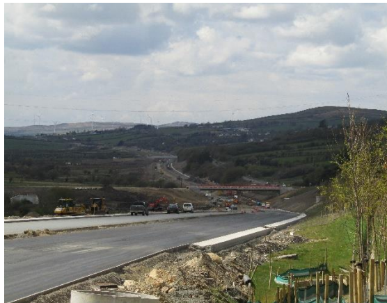
Construction of dual carriageway at Ballyhanedin.
