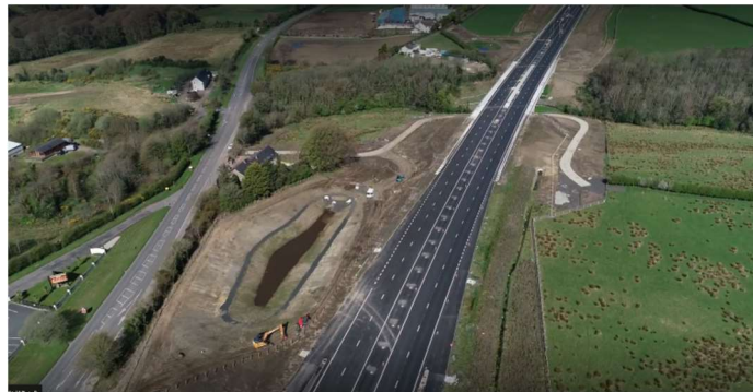
A6 Dual Carriageway at Liberty Glen
