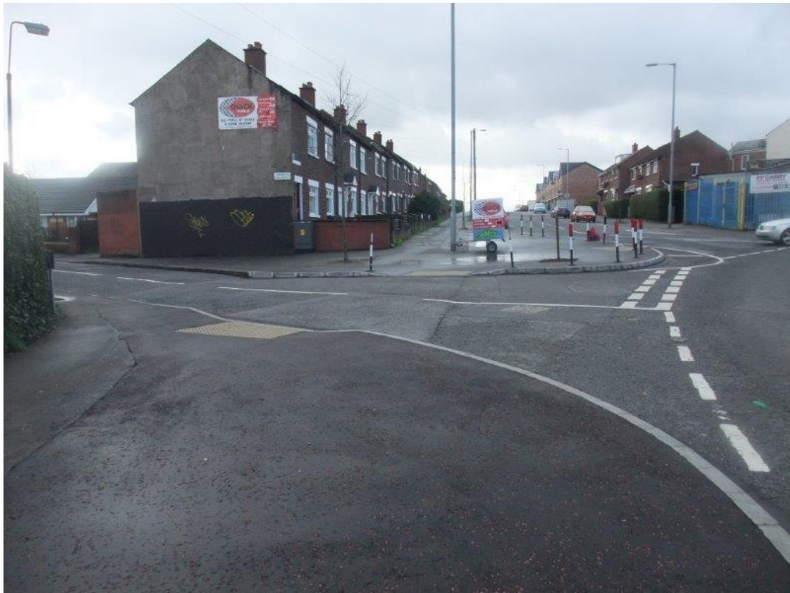
Oldpark Road at Torrens Avenue – junction improvement
