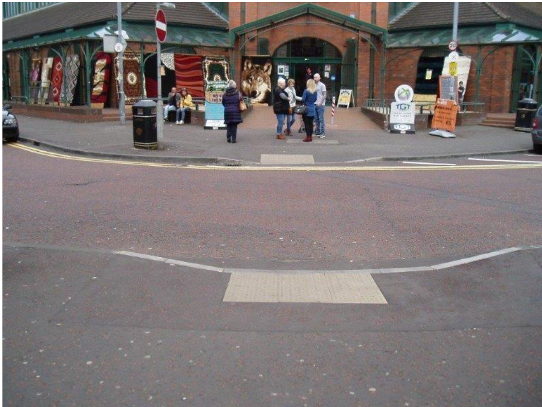
Smithfield Square – dropped kerbs and tactile paving
