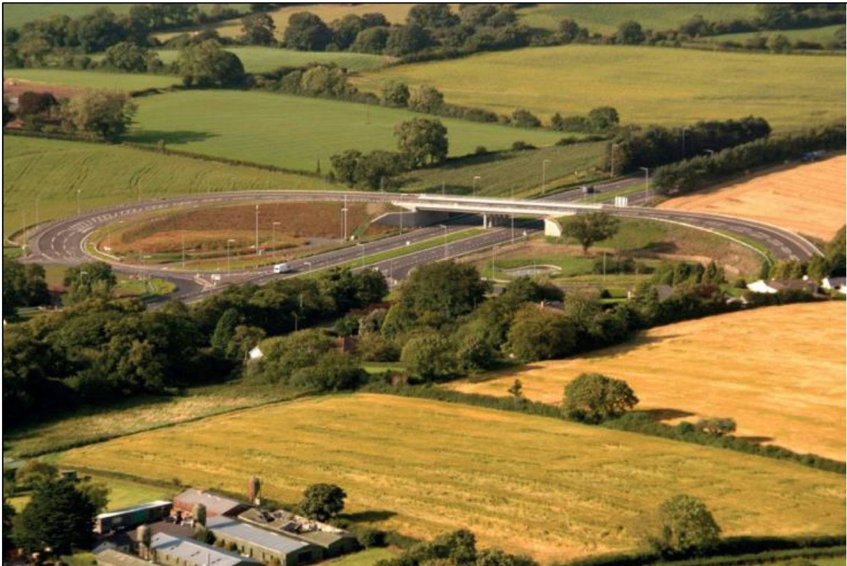
Existing Compact Grade Separated Junction at Pantridge Link, Hillsborough
