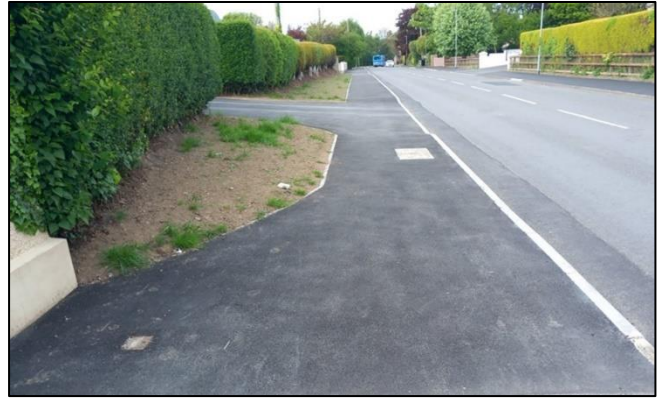
Provision of a new footway.
