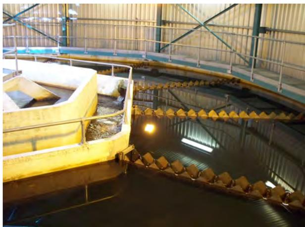
**Figure 2.2: Backwashing a Filter**
