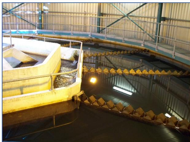
**Figure 2.2: Backwashing a Filter**
