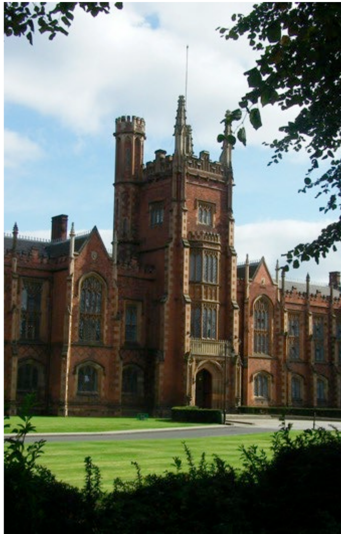
FIGURE 17. CENTRAL PORTION OF THE LANYON BUILDING, QUEEN'S UNIVERSITY BELFAST.
