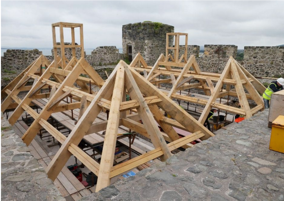
FIGURE 20. CARRICKFERGUS CASTLE, REPLACEMENT AUTHENTIC ROOF STRUCTURE
