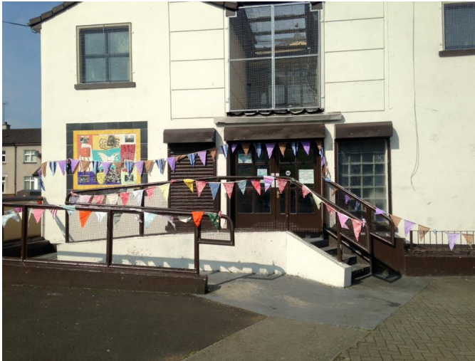
Dove House repainted outside
