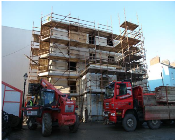
The Manse during the building phase of refurbishment
