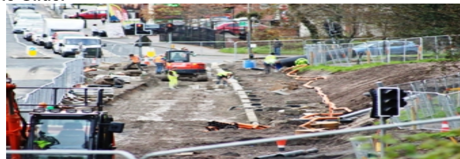
Ongoing road works to facilitate the Glider
