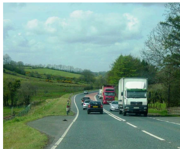
Traffic on the existing A5
