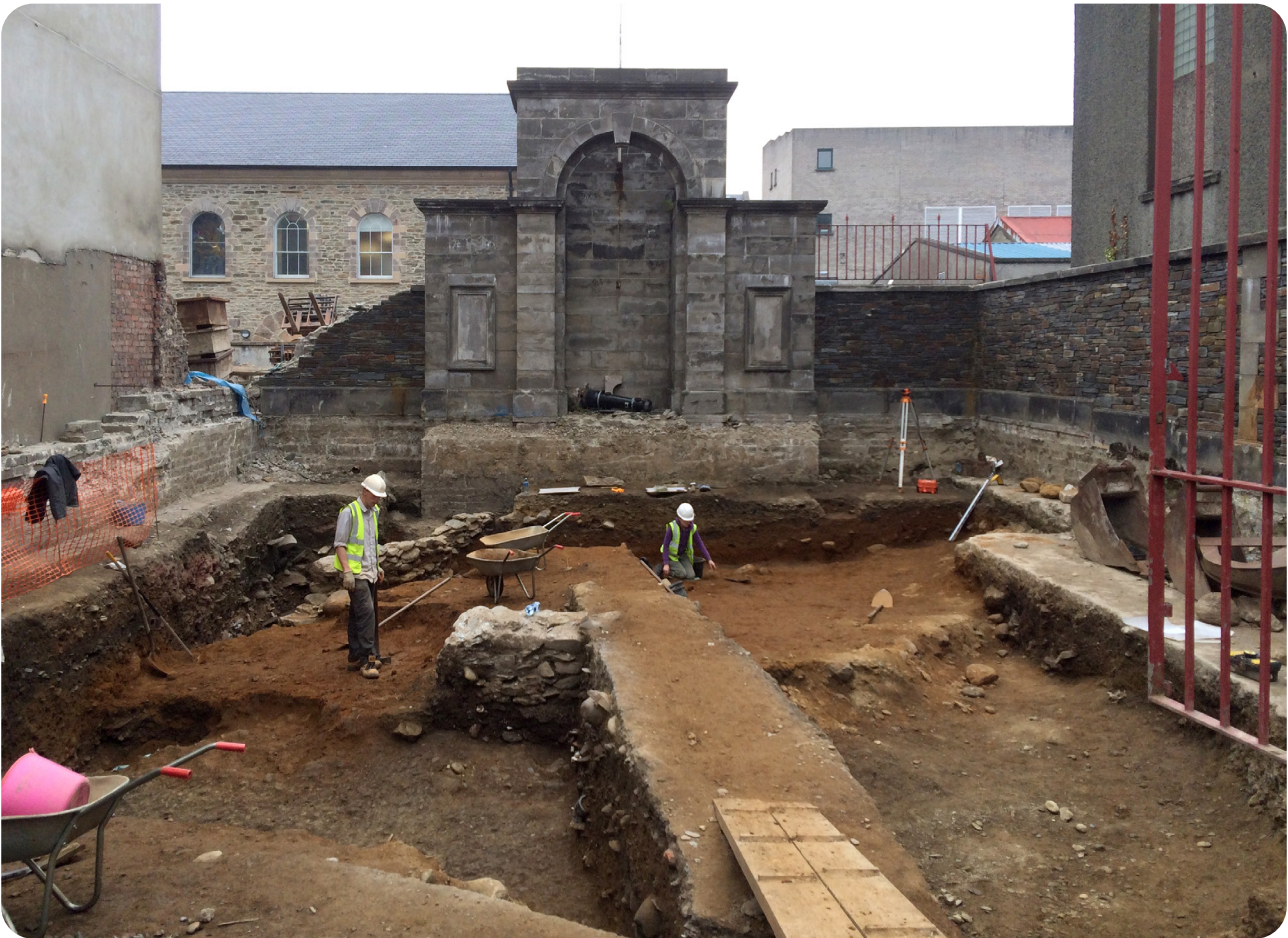
Excavations of medieval and post-medieval structures at Society Street, Derry/Londonderry
