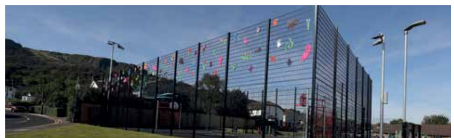
An open-mesh fence replaces the old peace fence with colourful artwork designed by local children.
