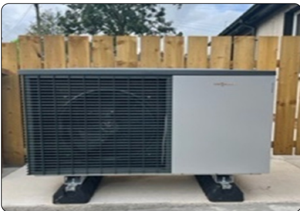
Air Source Heat Pump installation at Arbour Housing Association site in Banbridge.
