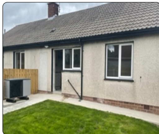
Air Source Heat Pump installation at Arbour Housing Association site in Banbridge.
