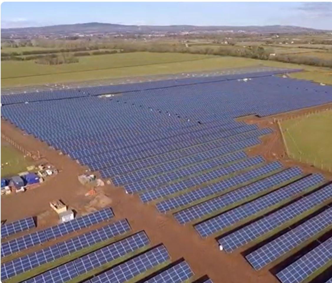
NI Water's investment in solar PV with battery storage at Dunore Point water treatment plant
