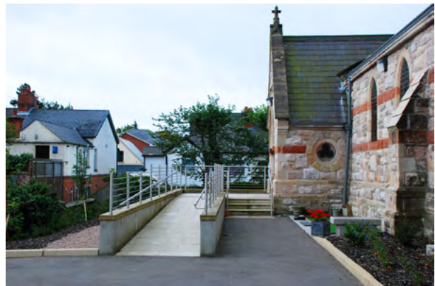
Example of adding to an historic building to make it accessible
