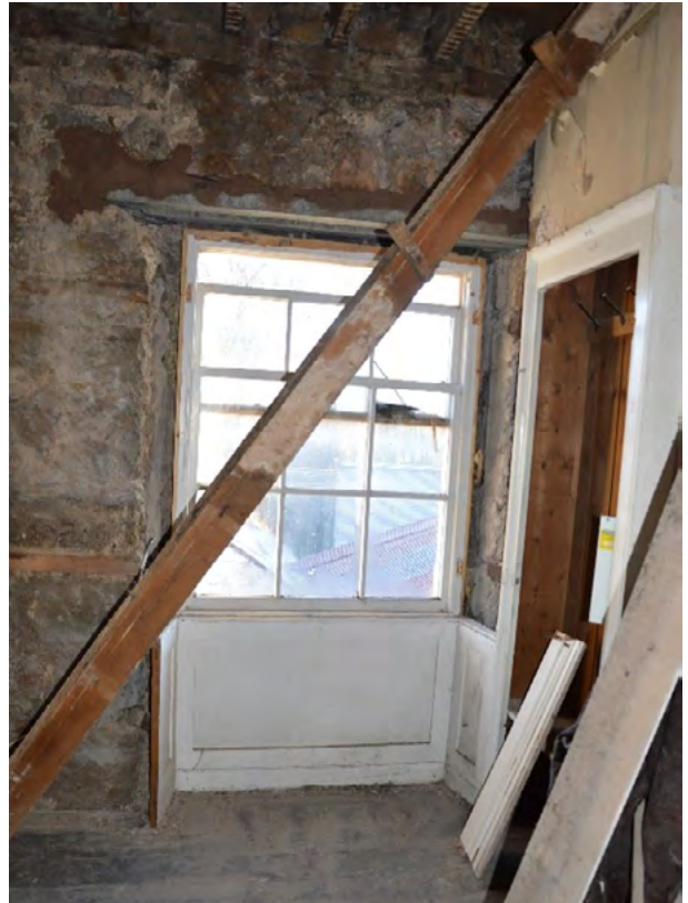
Removed window lining (left) and masonry reveals (right) - a difficult area to address when improving the thermal performance of the building
