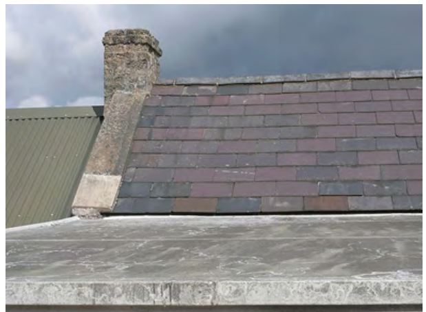
Slate roof with lead 'catslide' and modern corrugated roof abutting
