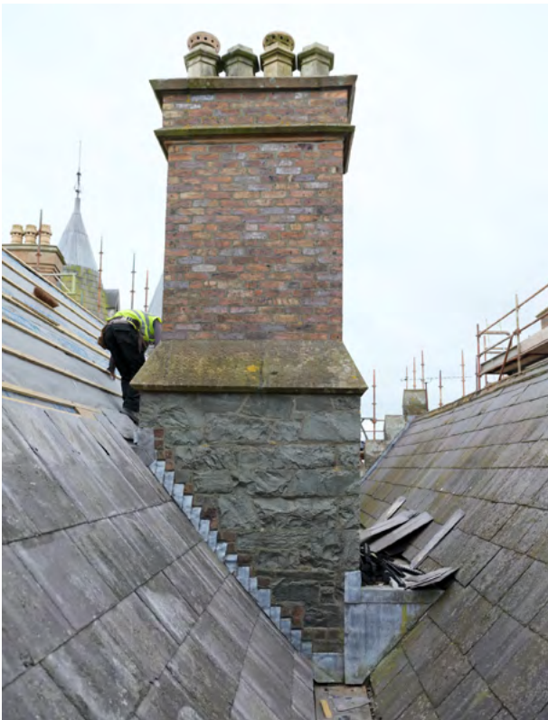
Valley to slate roof, double pile arrangement
