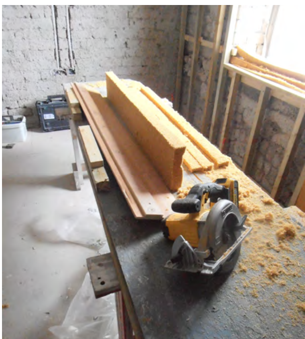
Wood fibre insulation on site
