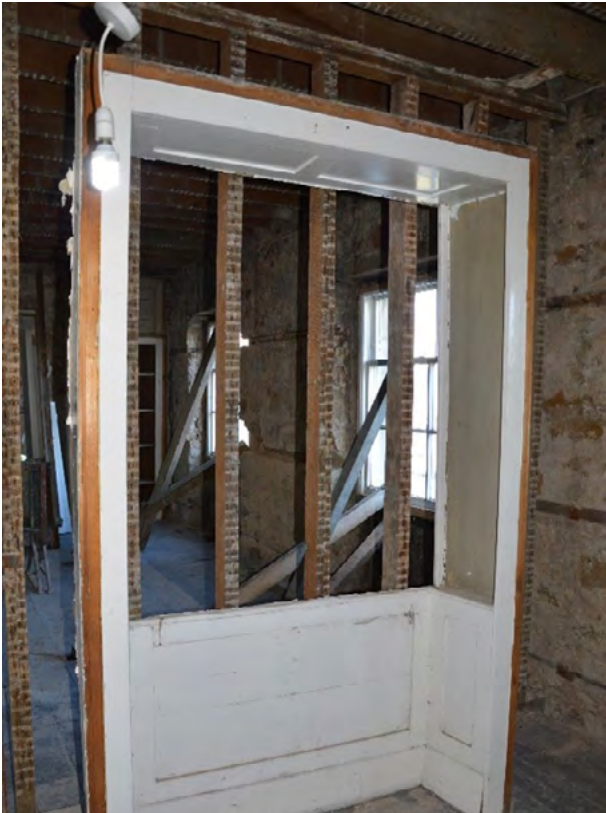
Removed window lining (left) and masonry reveals (right) - a difficult area to address when improving the thermal performance of the building
