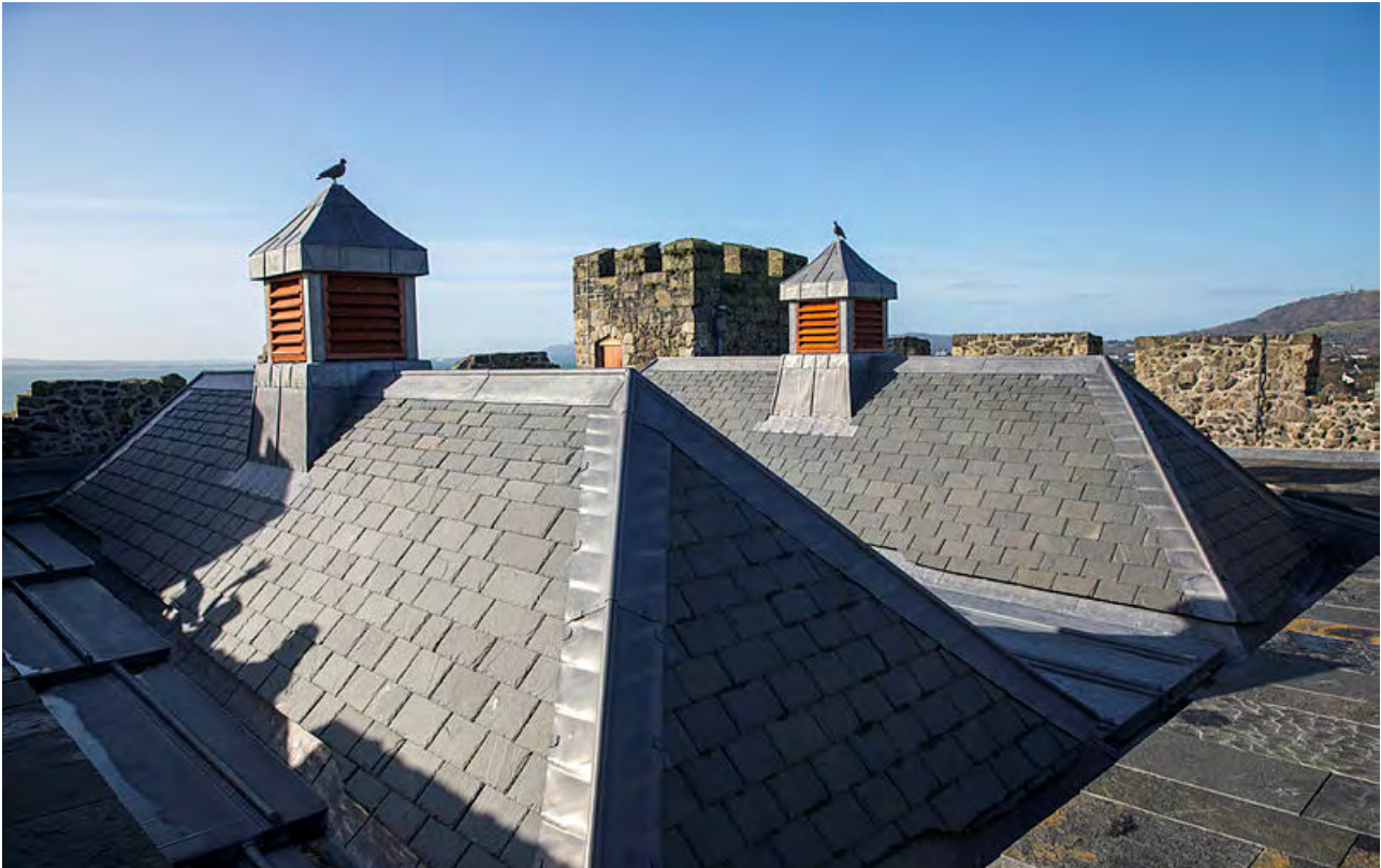
New double pile roof at Carrickfergus Castle
