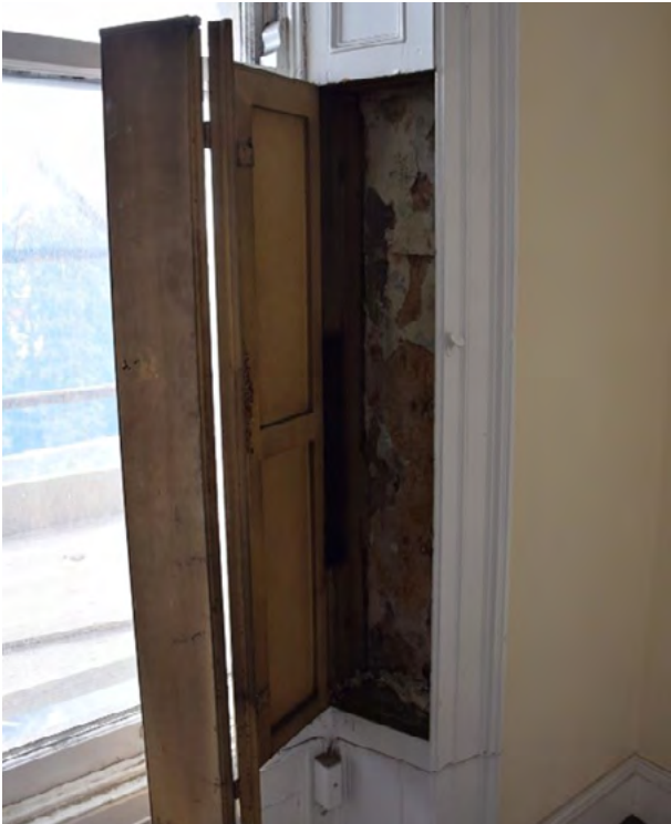
Shutters to reveals
