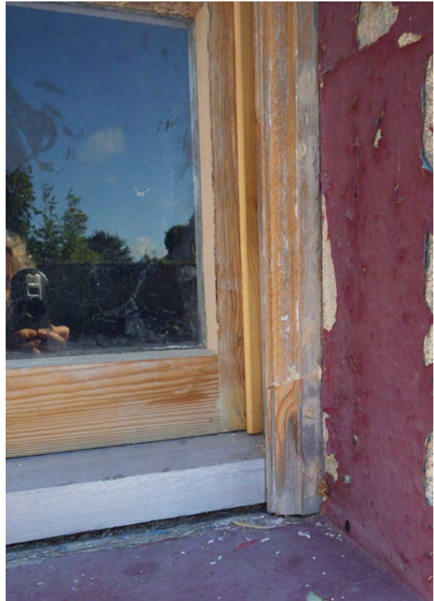
Repairs to window, timber cill, parting bead, putty and outer trim
