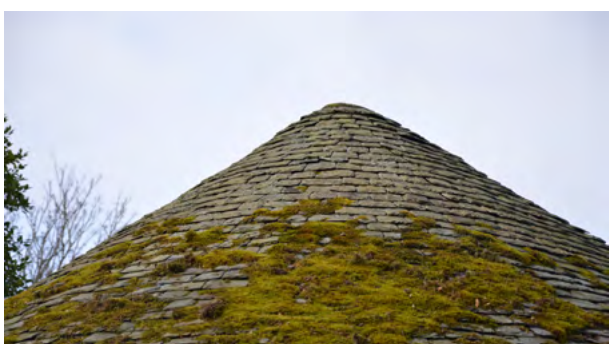
Tullycavey slate roof
