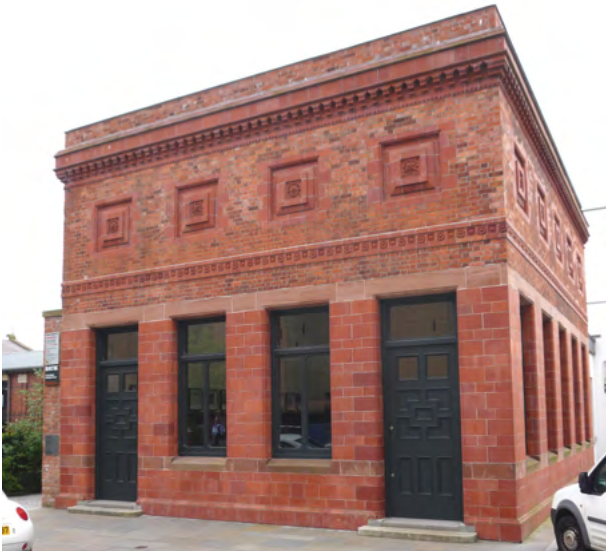
Belfast Gasworks Meter House
