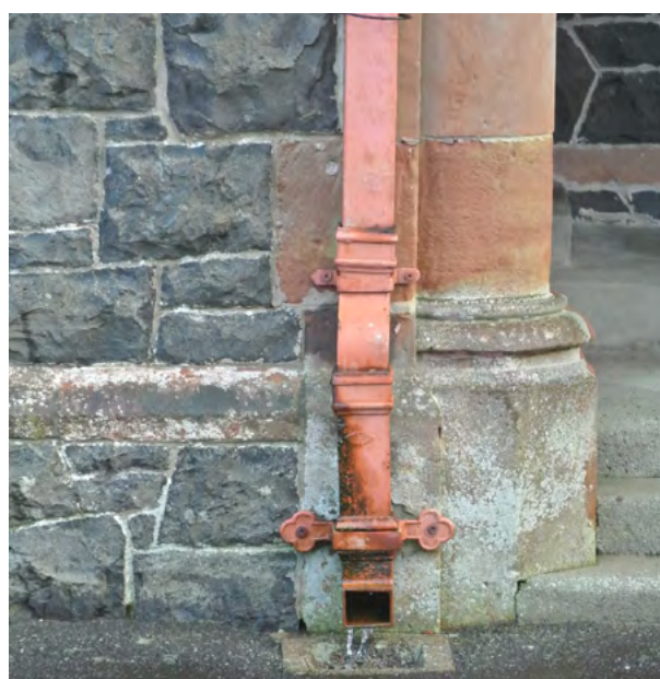
Cast iron downpipe discharging into gully and keeping the base of the wall dry
