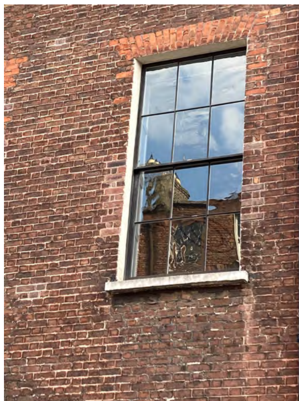
Historic Georgian window and glass
