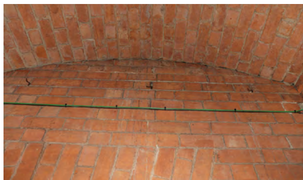
Brick barrel vault supported floor above,
