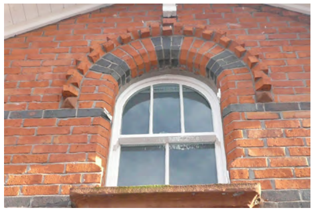
3 panes over 2 sliding sash timber
