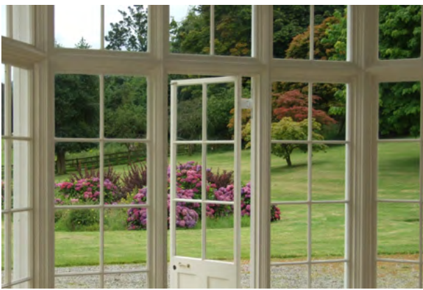
Bay window with door slim profile timber
