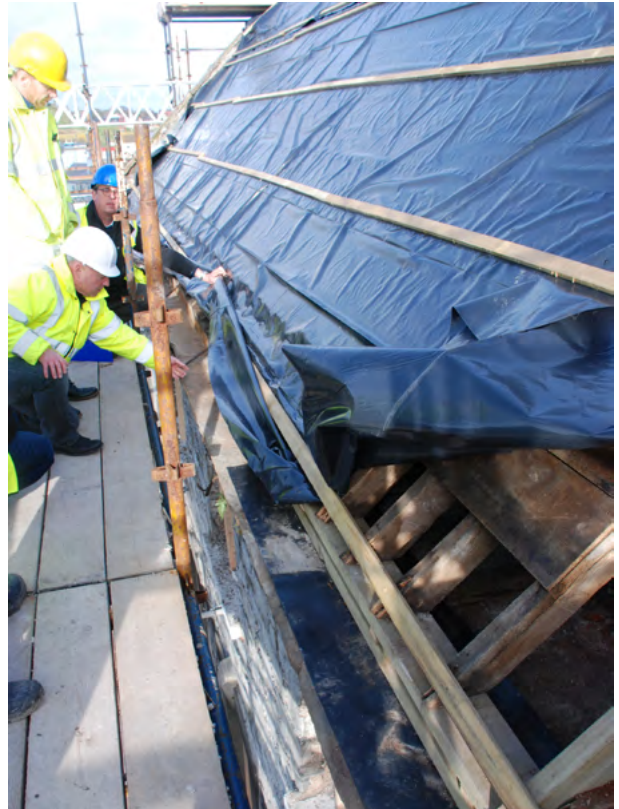
Sarking board under protective layer during build
