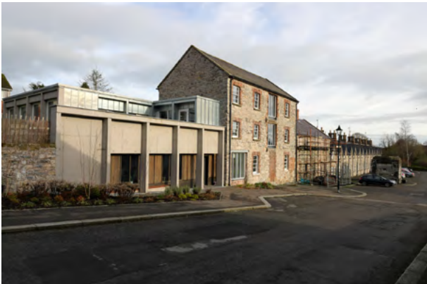
Caledon Wool Store with contemporary extension
