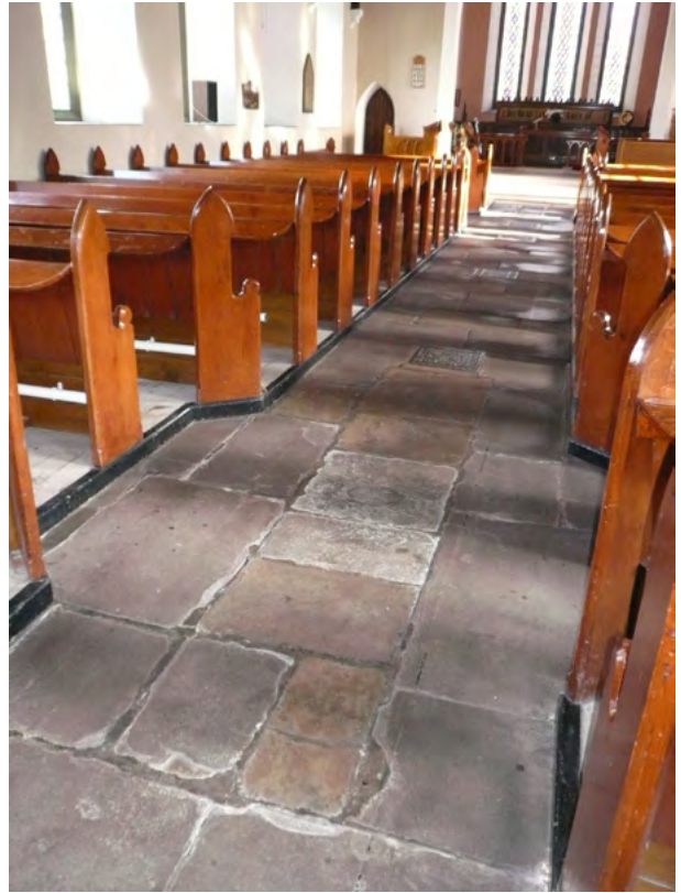
Stone flagging to church aisle
