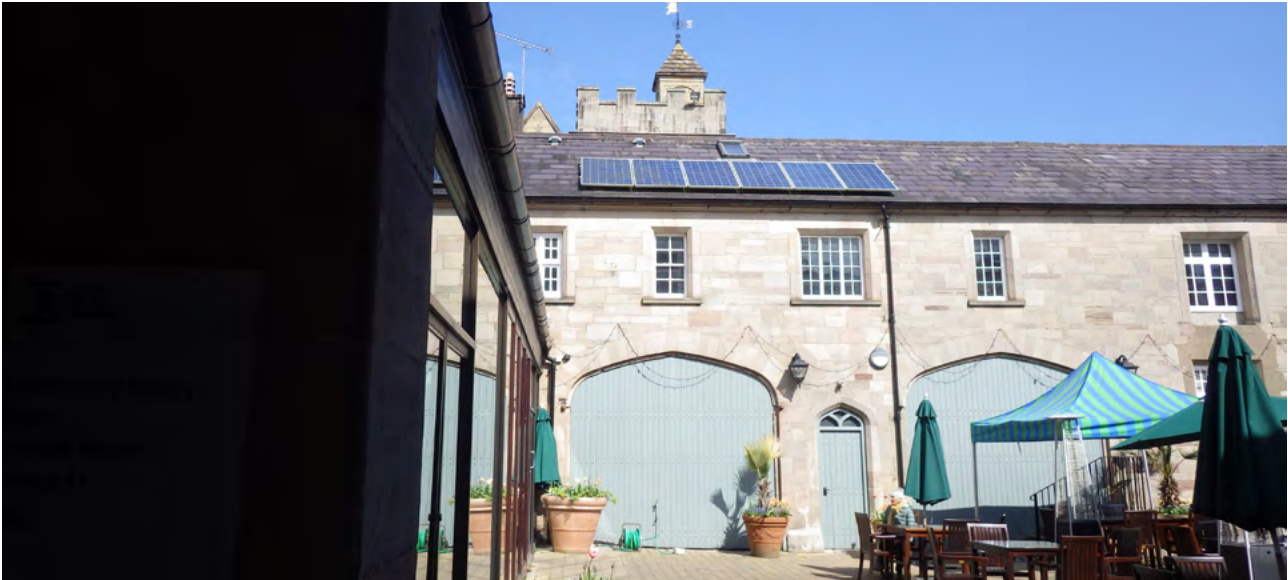
Photo voltaics in discreet location on inner courtyard roof
