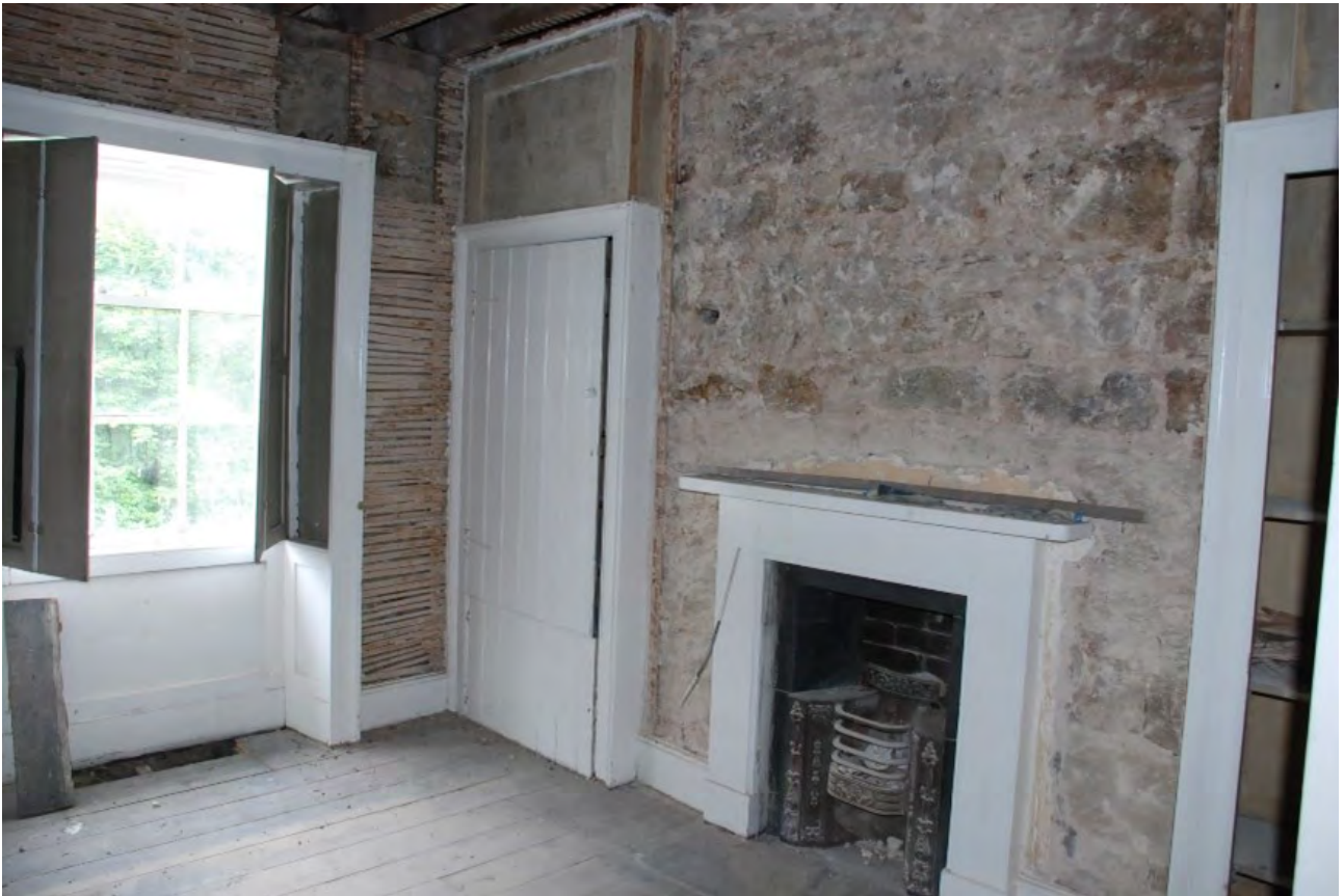
A number of fixtures and fittings to be considered if retrofitting: historic lath, built in cabinetry, window linings, shutters all present challenges for insulating internally and the level of removal or dismantling may not be feasible.
