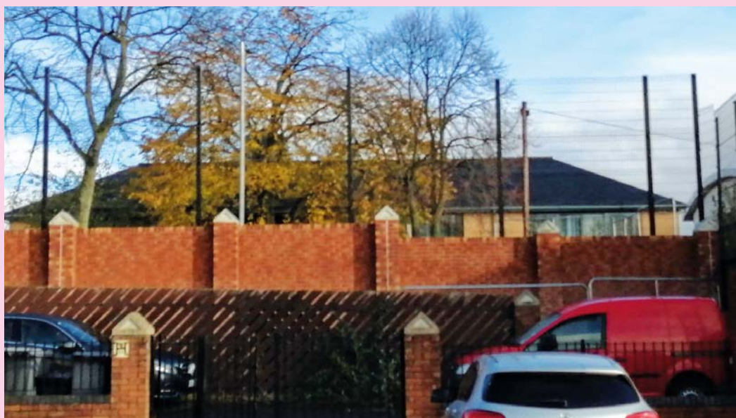
LEFT: Hillman court in North Belfast with new fencing.
