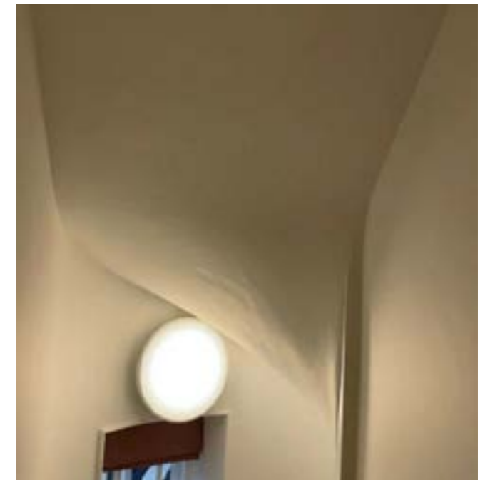
Ceiling finish with intumescent coating applied
