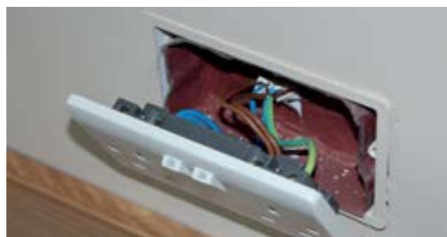
Double plug socket with intumescent gasket installed
