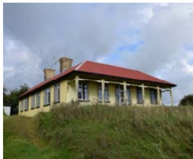
Darjeeling House, Enniskillen ( before demolition)
