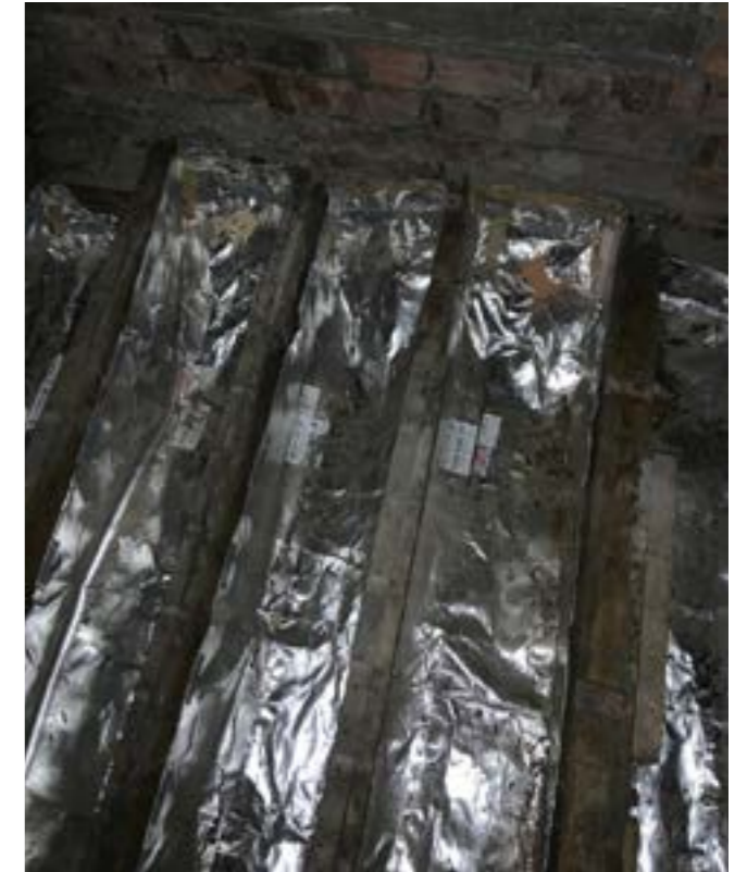
Floor rafters with insulation with intumescent coating barrier
