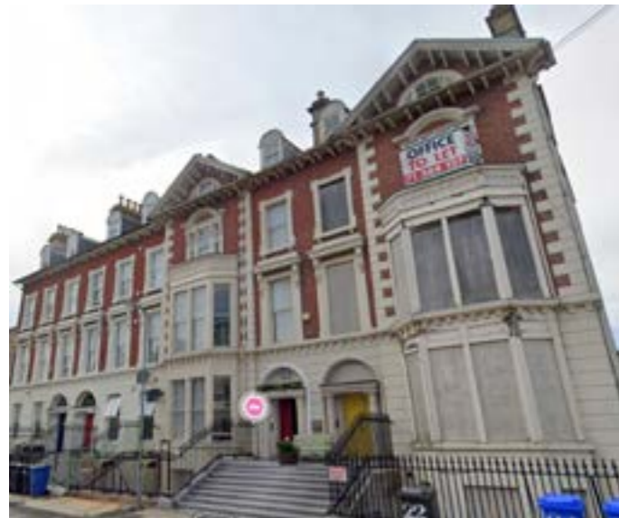
Refurbishment of listed building in Derry
