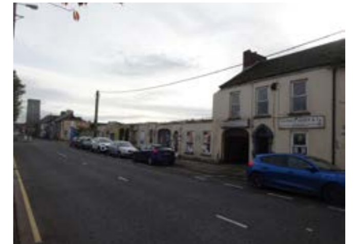
47-55 and 63-65 Court Street demolished, an unpleasant sight
