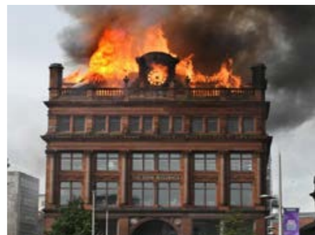
Fined £80K for Health & Safety Breach over Belfast Primark Fire
