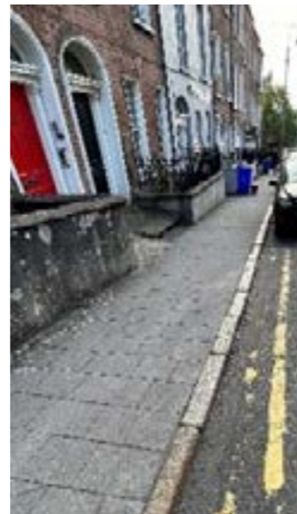
Granite kerb sets in Conservation Area
