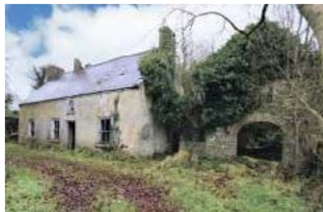
Former Manse, 36 Glen Hoy Road, Augher
