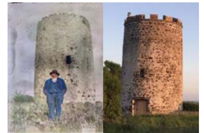
The Stump, Cockhill, Drumaphy, County Armagh - built as a windmill in c.1706 and owes its survival to conversion into a dwelling in c.1840. Photo of Mr Bill Totten outside his adapted historic home in c.1900. The building would not have survived had it not been for the acceptance of change but retention of character and a (then) culture of reuse rather than rebuild. Today The Stump consists of three building phases yet we see it as one heritage building, with each part of its narrative adding to its interest (Image source: own).
