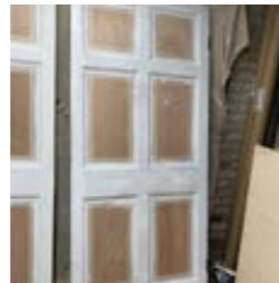
Timber door showing intumescent card and coating upgrade in progress
