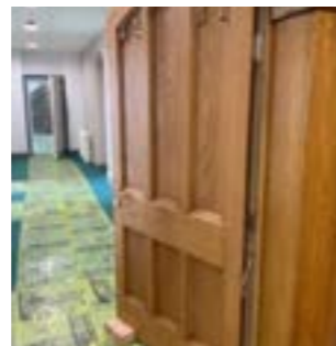
Door upgrade at Methodist College, Belfast
