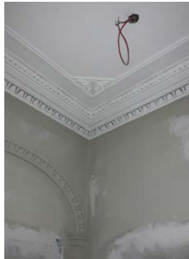
Cornice detail with intumescent coating applied
