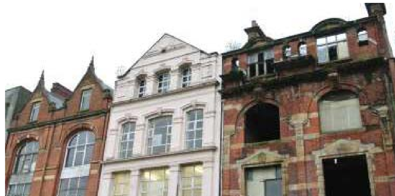
Three 'nearly listed' buildings on Belfast's North Street in 2016, before demolition
