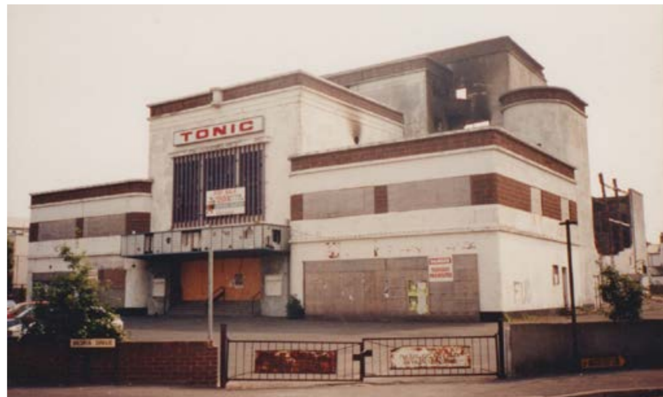
Tonic Cinema following major fire damage, 1992. Courtesy Gary Cosby
