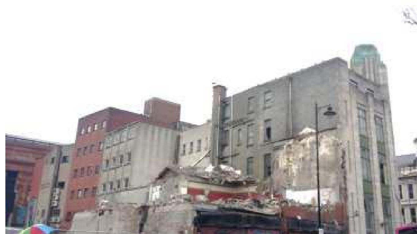
The same buildings after demolition
